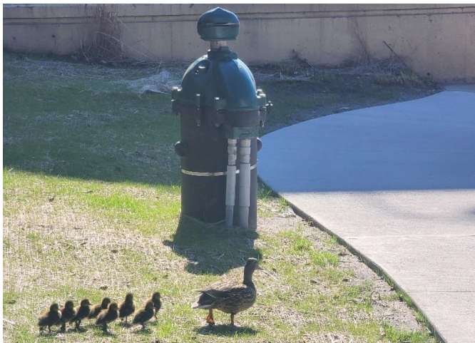
Geothermal well installation at Rochester city hall
